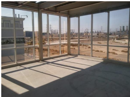
The Property – Internal view
