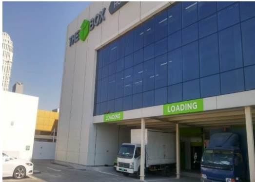
The Property – Exterior View
