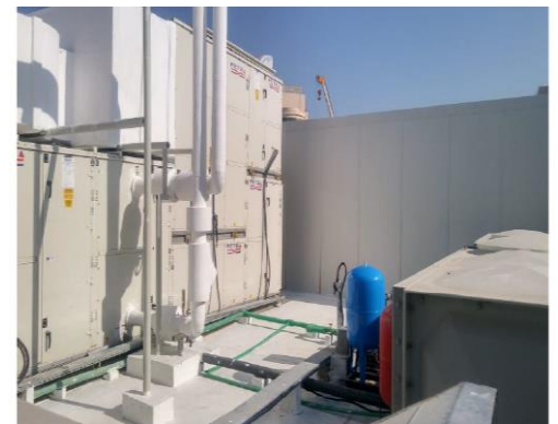
The Property – Roof
